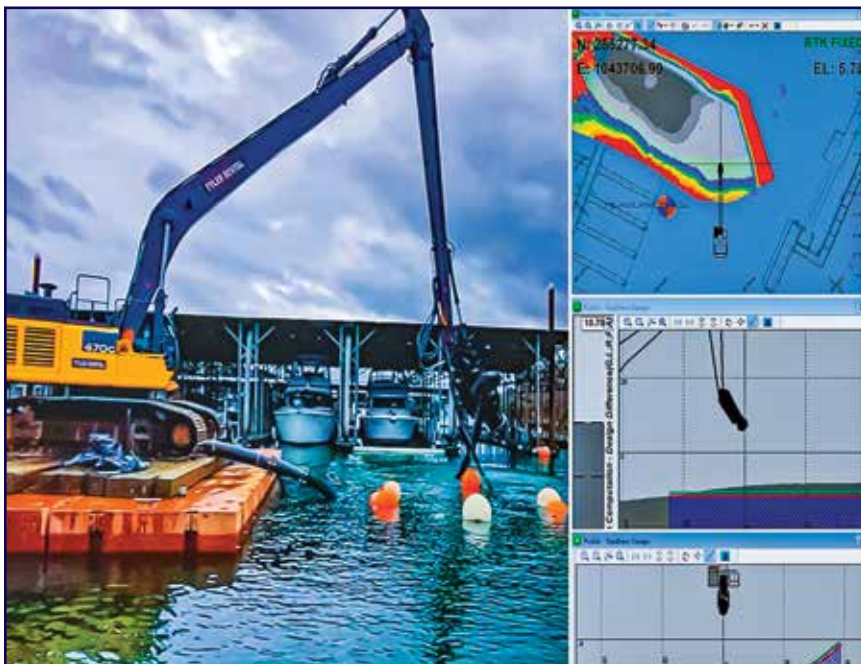
Trimble Marine Construction software provides the operator with plan and profile views to ensure accuracy
