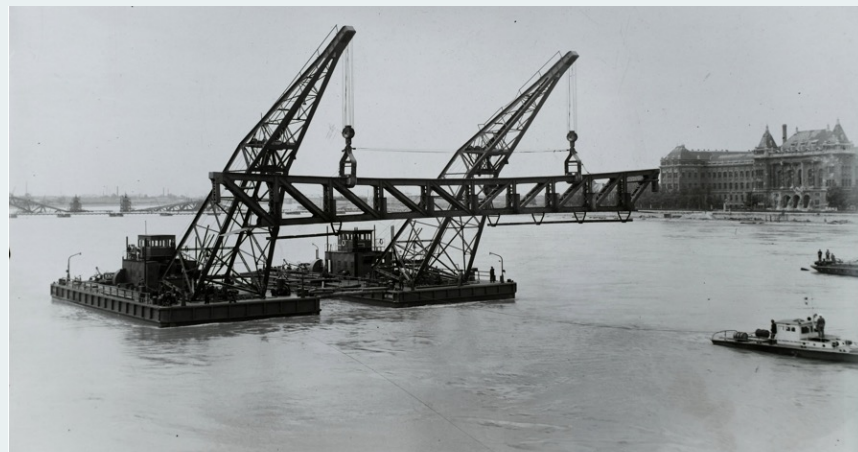
Construction of the central part of the bridge on 12 July 1946 (Source: Fortepan / Hungarian Museum of Technology and Transport / Collection of Historical Photographs / Ganz Collection / TFGY 2017.1.1105)
