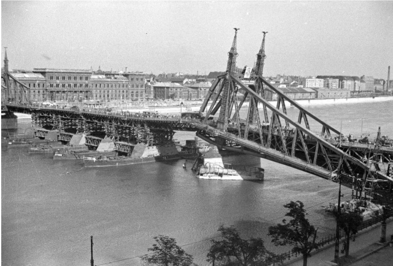
Liberty (former Ferenc József) Bridge during reconstruction
