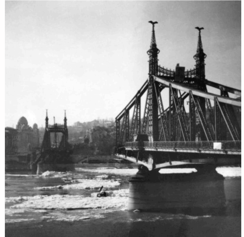
Liberty Bridge after destruction in 1945, showing the center section destroyed. Image credit: Wikimedia Commons.
